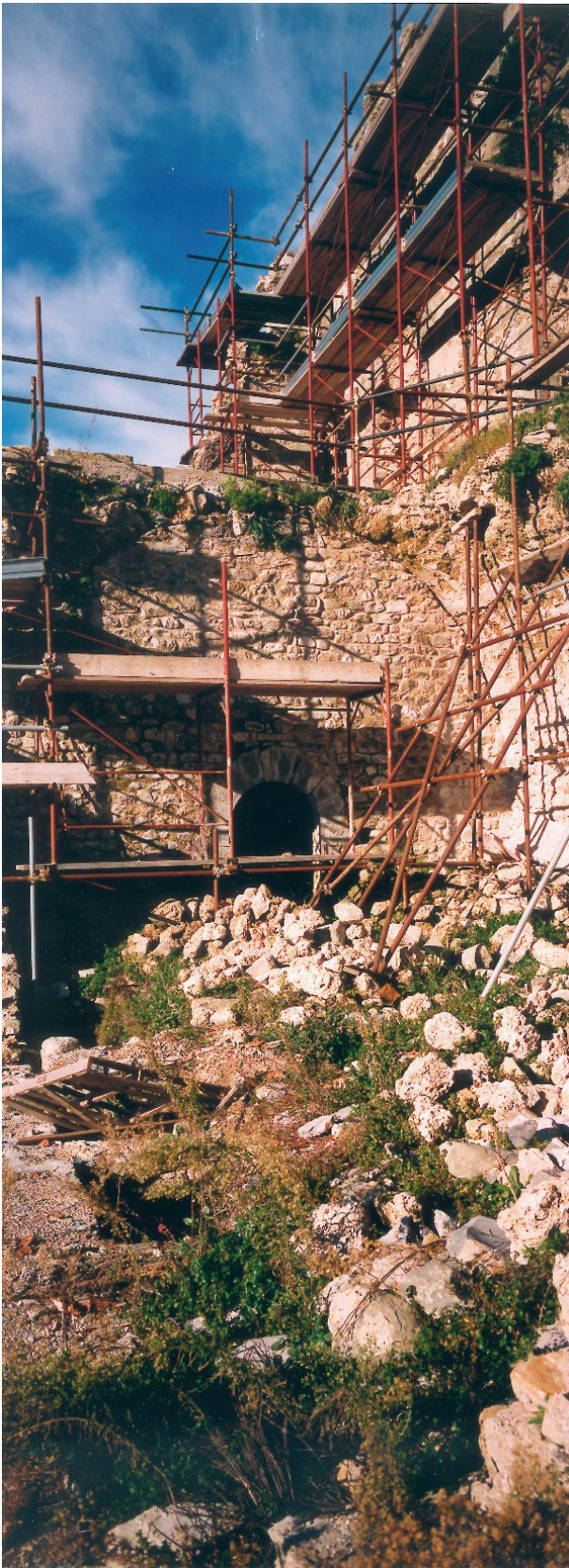
Fig. 6. The main room of the south wing during excavation. Image by the author.
