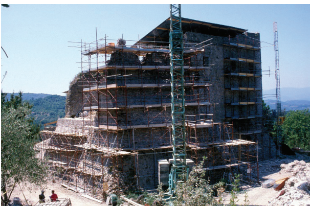
Fig. 16. The very image of the keep with the scaffolding that primed the idea for the proposed solution for its reconstruction. Image by the author.
