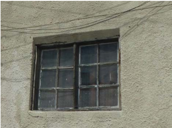
Fig. 15. A typical steel window. Image by Bahrain Authority for Culture and Antiquities.
