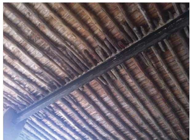
Fig. 8. Steel beam replacing a dividing wall in order to join two storage spaces together, in the Muharraq Suq. Image by Bahrain Authority for Culture and Antiquities.
