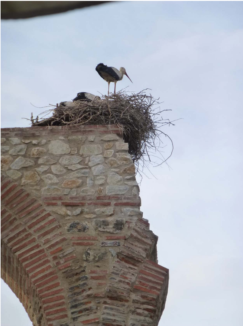
Fig. 4. Roman aqueduct and pelicans nesting, Selcuk Municipality, Turkey. Image by the authors.
