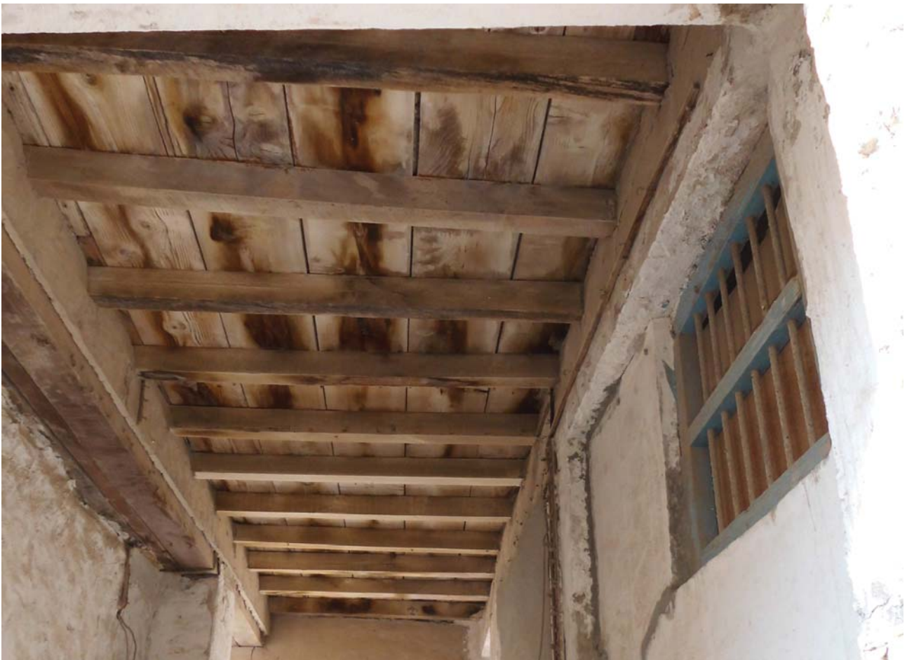
Fig. 11. The new construction system using square wooden beams and ply-wood. Image by Bahrain Authority for Culture and Antiquities.
