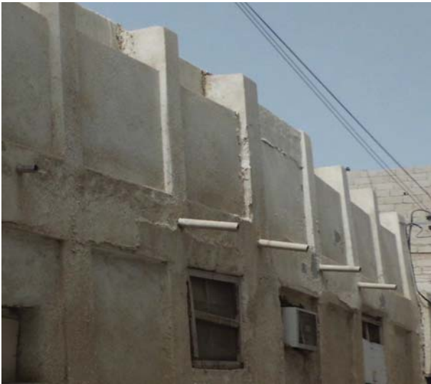
Fig. 17. Series of niches and badgeer made of block work, the niches are only 5 cm deep. Image by Bahrain Authority for Culture and Antiquities.
