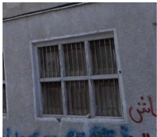
Fig. 18. A rare example of a wooden window with iron bars (traditional) mimicking the steel windows of the transitional style. Image by Bahrain Authority for Culture and Antiquities.
