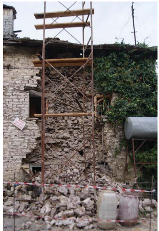
Fig. 5 & 6. A portion of the Hadëri house in 2014 (left), two years after a devastating fire. One wall of the Gurgai house (right) collapsed in 2014 after a heavy rain. Images by CHWB.
