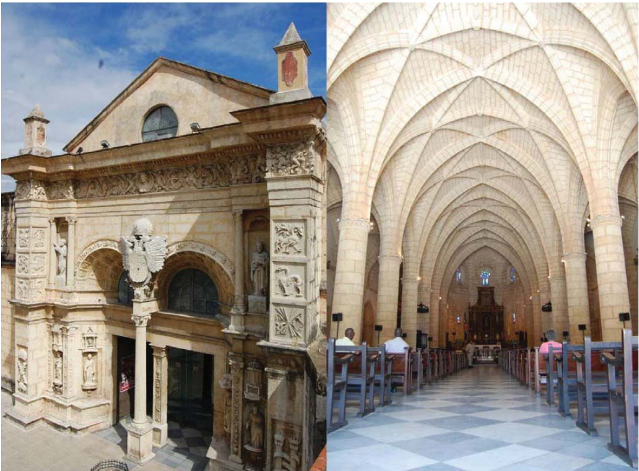
Fig. 16. Restoration Results. Façade and Interior , 2010 (Courtesy of Esteban Prieto).
