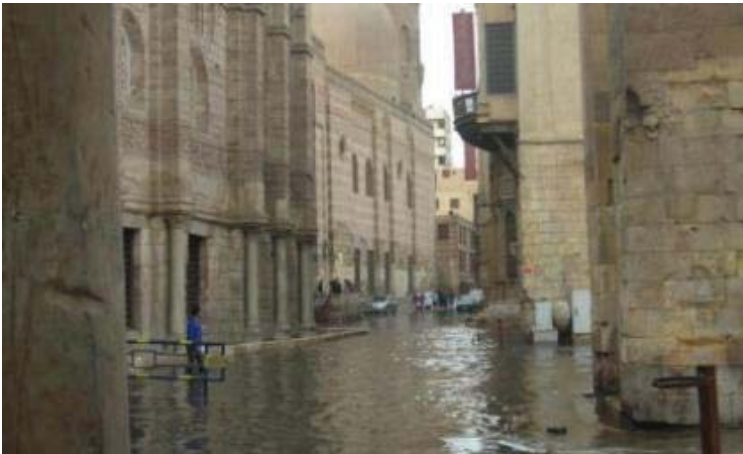
Fig. 5. The Muezz street flooded by the sewage water (El Badil website).
