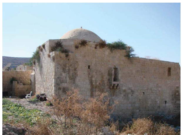
Fig. 4. 'Abwein village. Dar Sehwil, Eastern restored external wall. Ramallah, Palestine.
