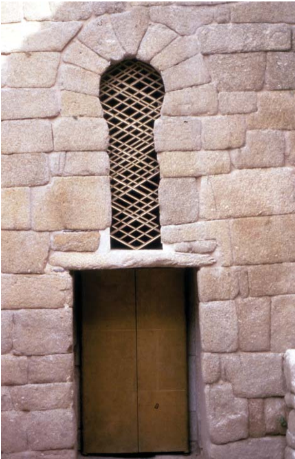
Fig. 6. New grille in the church of Santa María de Melque. The metal rods indicate all the previous holes from preceding grilles.
