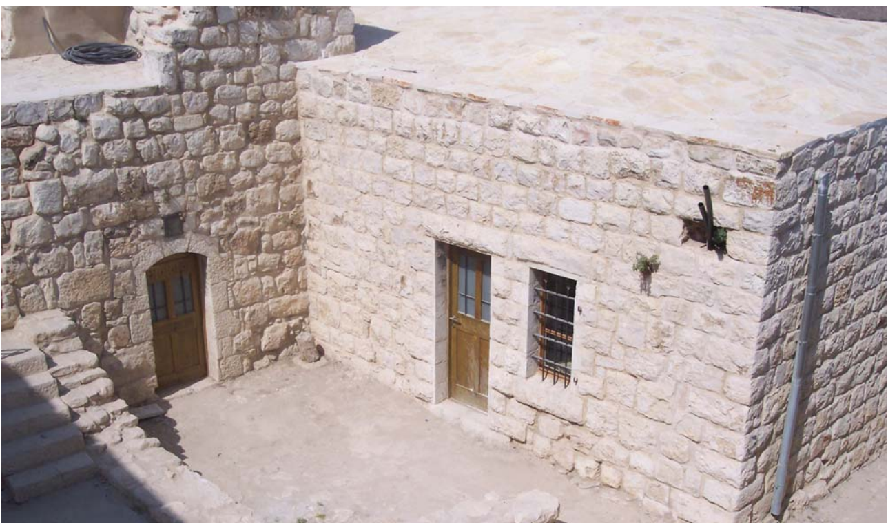
Fig. 7. Et-Taiyiba village. General view of the restored houses. Ramallah, Palestine.
