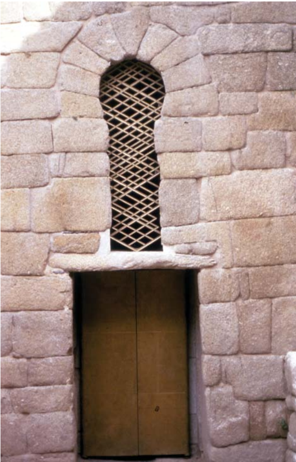
Fig. 6. New grille in the church of Santa María de Melque. The metal rods indicate all the previous holes from preceding grilles.
