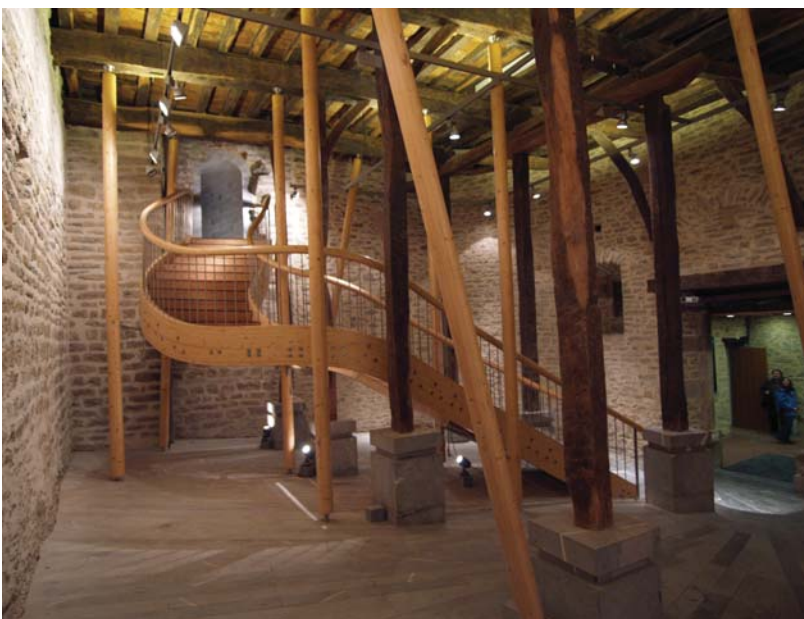
Fig. 9. New stairs to access to the Cathedral of Santa María de Vitoria, Spain. Restoration project by Latorre y Camara, arquitectos.
